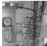
Electric and Gas Utilities
