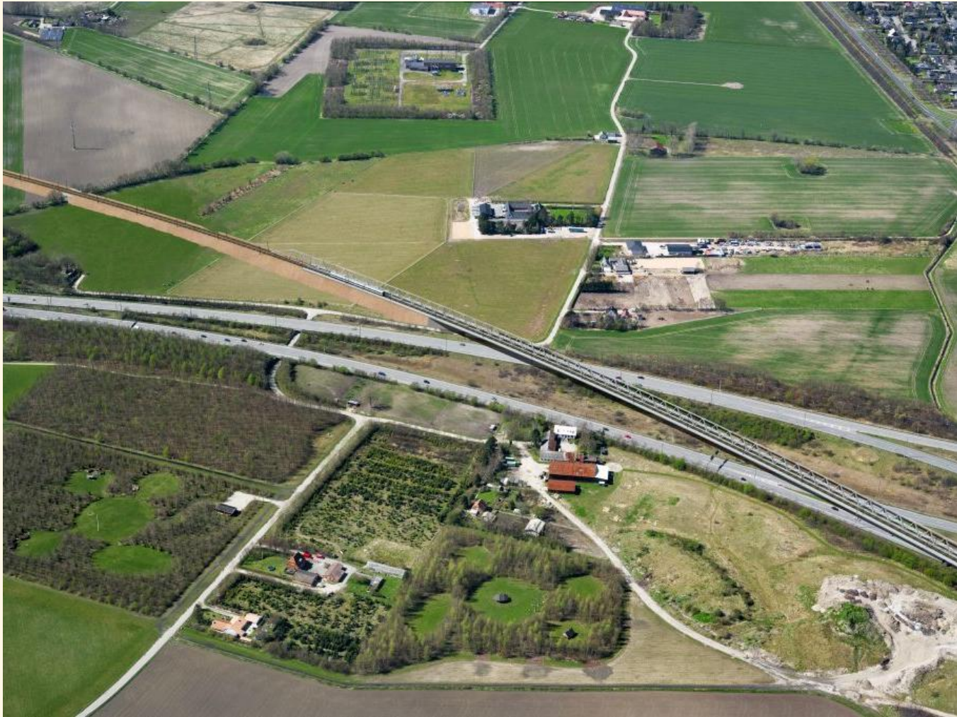
Long bridge over M-way
